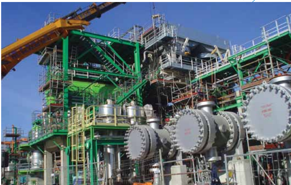
2005 / FRANCE Piping Erection for TOTAL Refinery - La Mede
