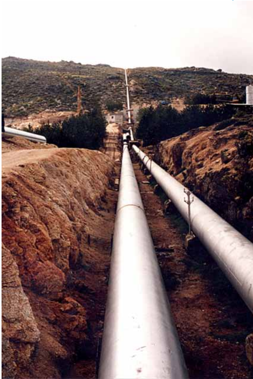
1992 / SERRA DA ESTRELA - PORTUGAL Erection of Forced Duct
