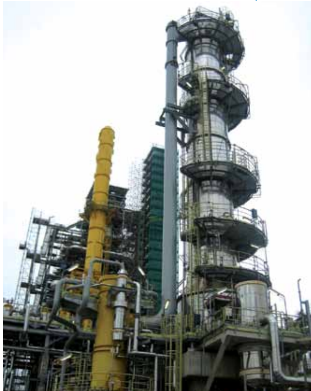
2008 / GONFREVILLE - FRANCE Piping Erection for TOTAL Refinery
