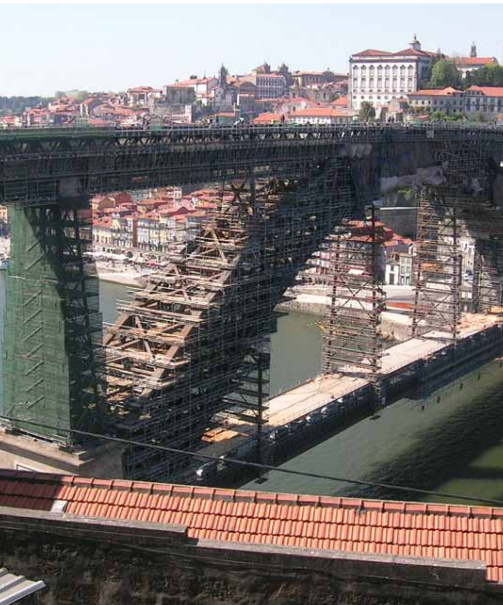
2004 / PORTO - PORTUGAL Reparation and Reinforcement of Steel Structures for D.Luiz I Bridge
