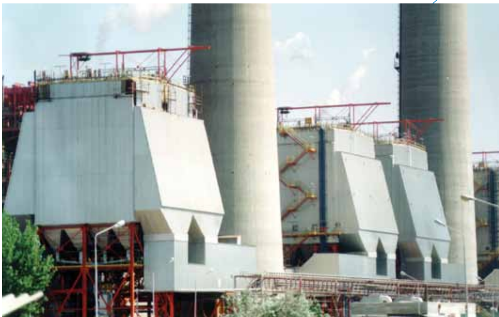
2001 / SETÚBAL - PORTUGAL Assembling of four Electrostatic Precipitators for EDP Power Plant
