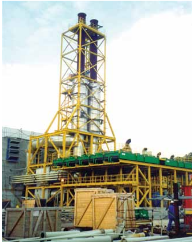
2001 / AZORES - PORTUGAL Mechanical Erection (Equipment and Piping) for Caldeirão Power Plant
