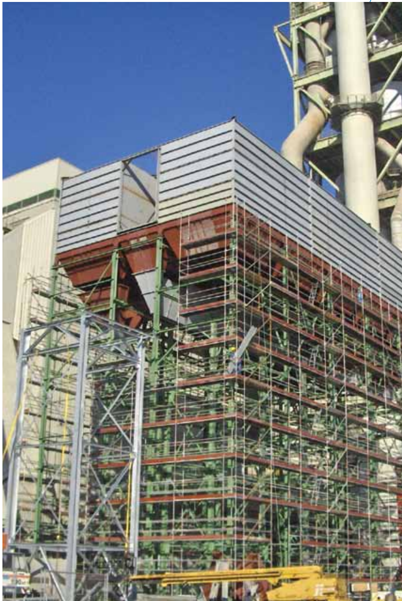
2005 / FRANCE Equipment Erection and Electrostatic Precipitator Repair for LAFARGE Cement Plant
